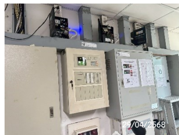
Fire Alarm Control Panel
